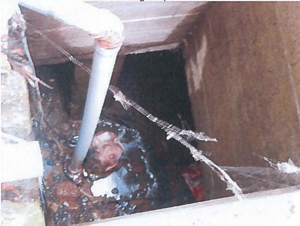
26. Drainage on eastern side of Grain Elevator building.
