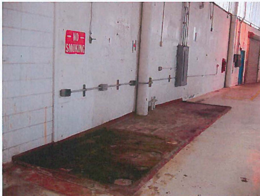
14. Interior of New Warehouse building, forklift charge area.
