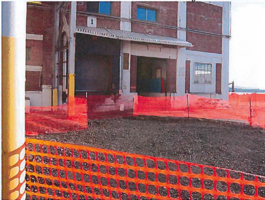
18. Former UST T-5 area, north Old Warehouse and Mill building, view to the southwest.
