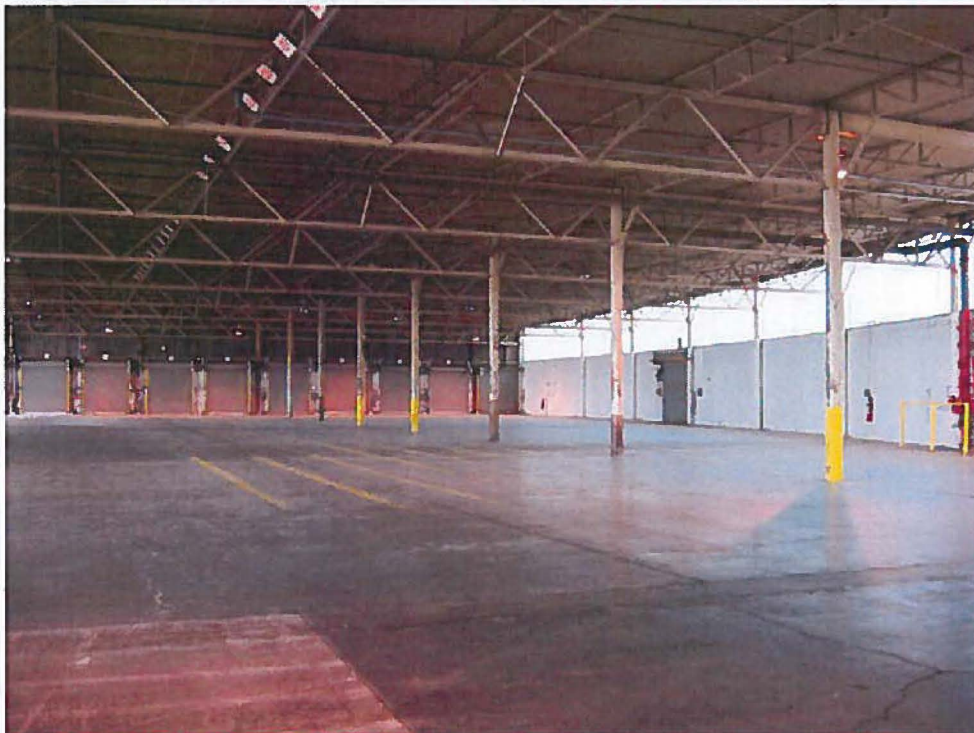
12. Interior of New Warehouse building.
