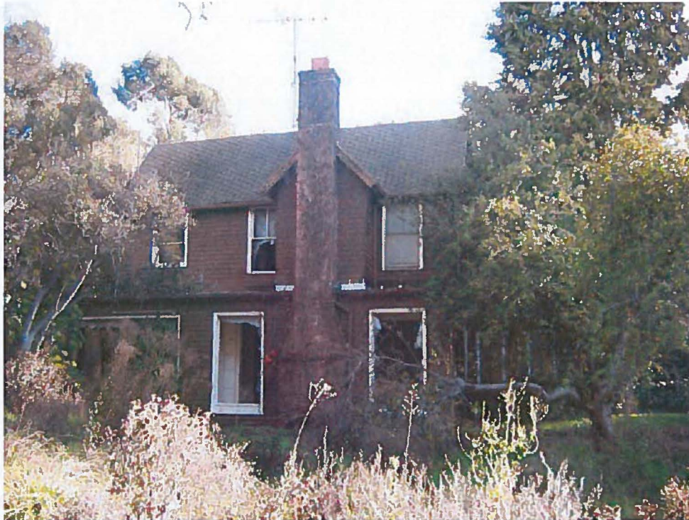
9. Plant residence, view to the east.
