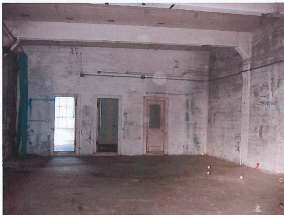
8. Interior of Garage building.
