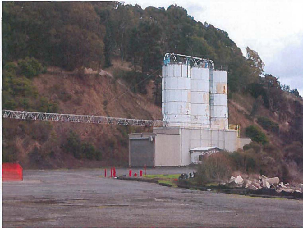
5. Mill run building on southern portion of the Site, view to southeast
