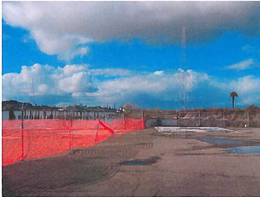
13. Former UST area T-1, T-3, T-4, and former AST area AST-4 and AST-5, northwest of the New Warehouse building, view to the northwest.
